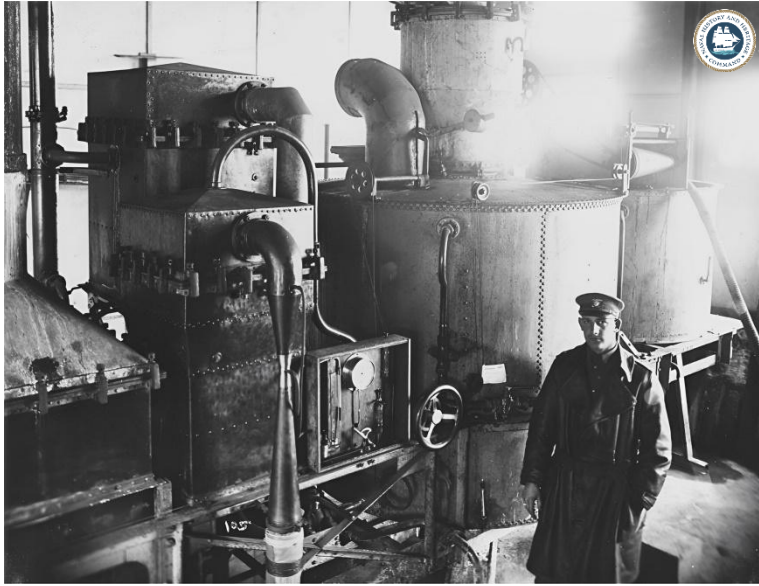
Installation semi-portable de 600 m 3 /h
